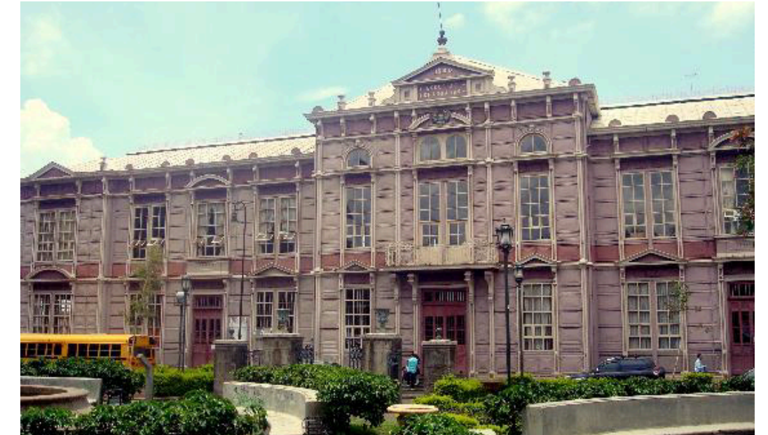
Escuela Buenaventura Corrales, also known as the Metallic Building or Metallic School, established in 1896.
